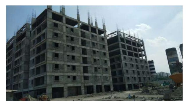
Block C2: Columns upto Ninth floor level 75% completed and balance works on progress. Slab Shuttering works at First half of Ninth Floor level 25% completed.
