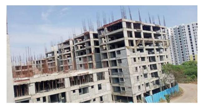
Block D3: Seventh Floor level slab First half concrete casting 100% completed. Barbending works for Second half of Seventh floor level slab on progress.
