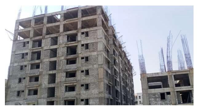
Block B2: Third Floor Level slab concrete casting 100% completed. Bar bending works for Columns up to fourth floor level on progress.
