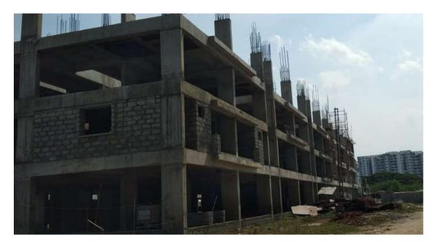
Block A2: Second Floor Level slab concrete casting 100% completed. Columns up to Third floor level 40% completed and balance work on progress
