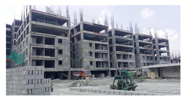
Block D1: Fourth Floor level slab First half concrete 100% completed. Slab shuttering works for second half of Fourth floor level 30 % completed and balance works on progress.
